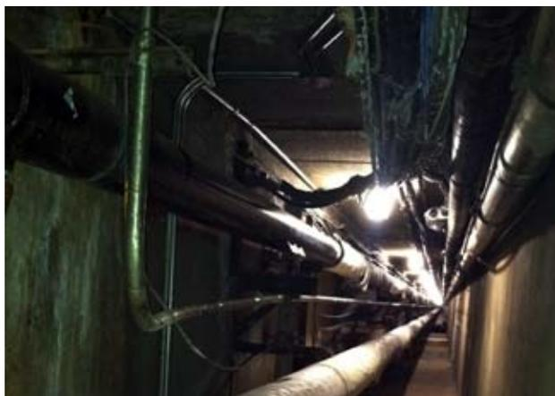
*Nearly six miles of insulation was installed on the steam lines, condensate lines, and chilled water supply and return lines in Weber State buildings in 2010. Projects like these help to keep the efficiency of the pipe system high*
