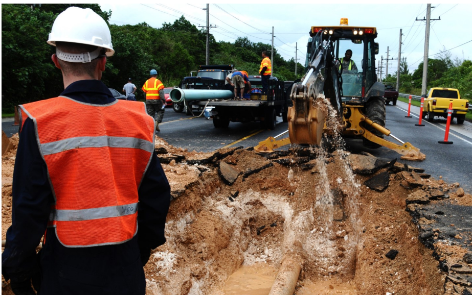
Road Demolition to change a section of a water main.
