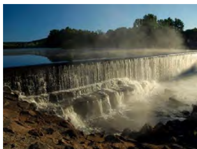
Eagleville Dam (Credit: Pinterest)
