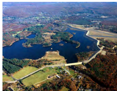
Mansfield Hollow Dam (Credit: ACOE)
