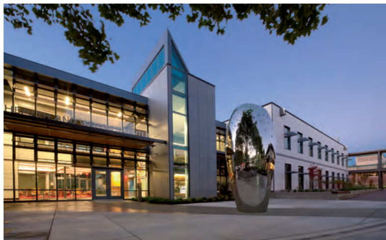
Lane Community College – Health & Wellness Center. Large projects funded by GRFs can generate a high volume of savings while providing a visible symbol of an institution's commitment to sustainability.
